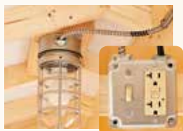
Electric Package Switch / Outlet / Lights Extension Cord Hookup
