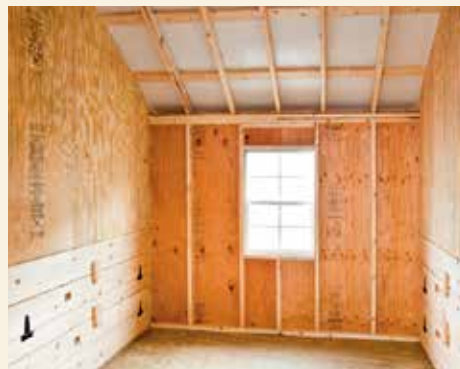
Feed room of A124 (shown above)
